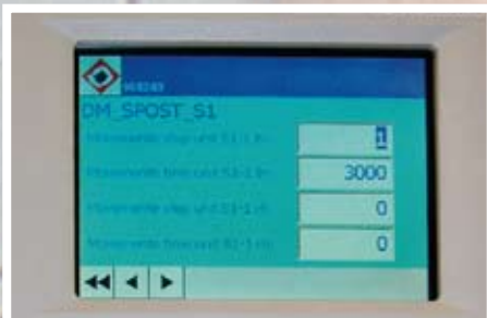
"Touch-screen" control panel.
